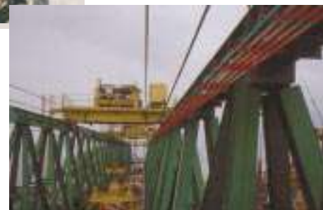
Bridge Construction Crane
