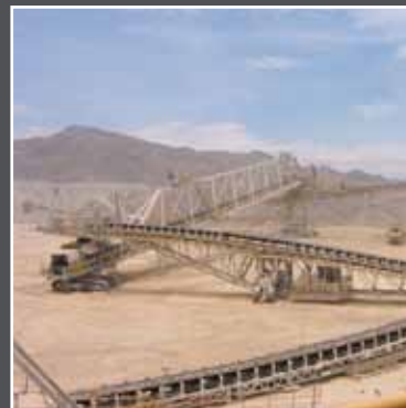
Festoon System on a Traveling Hopper, Peru
