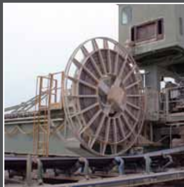
Level Wind Reel on a Stacker/Reclaimer, USA
