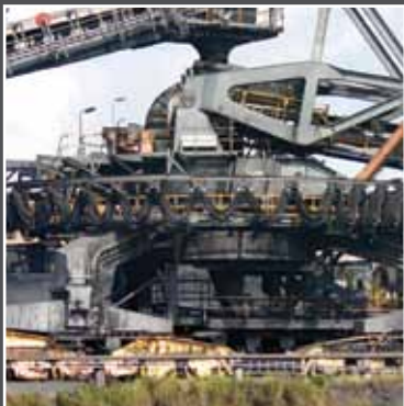
Festoon System on a Stacker/Reclaimer, Australia
