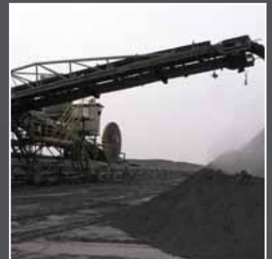
Motor Driven Cable Reel on a Stacker, Czech Republic
