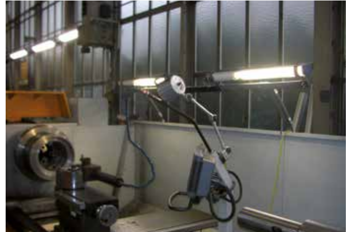
Workplace illumination, power plant
