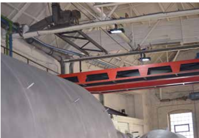
Corrosion protection industry
