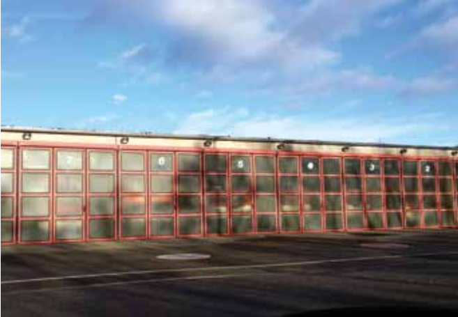
Illumination of equipment rooms, company fire brigade
