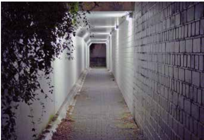
Underpass street lighting
