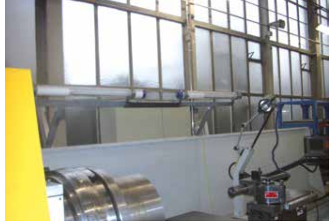
MasterLED - lathe workplace illumination
