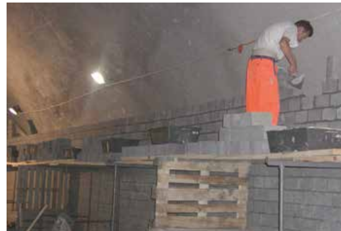
MULTI work light
