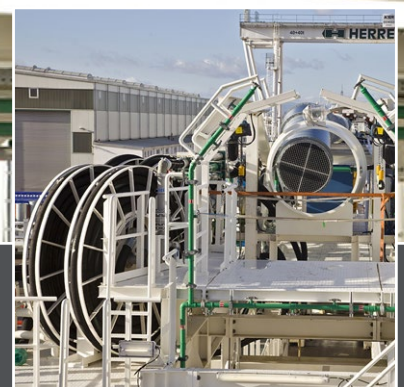
Hose reel during TBM build up for Herrenknecht "Rastatt" - Germany
