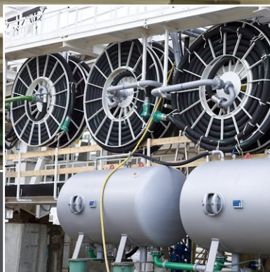
Hose reel during TBM build up for Herrenknecht "Bossertunnel" - Germany
